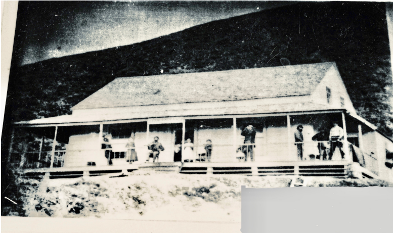
Tokatoka pub build by Capt. Stanaway
