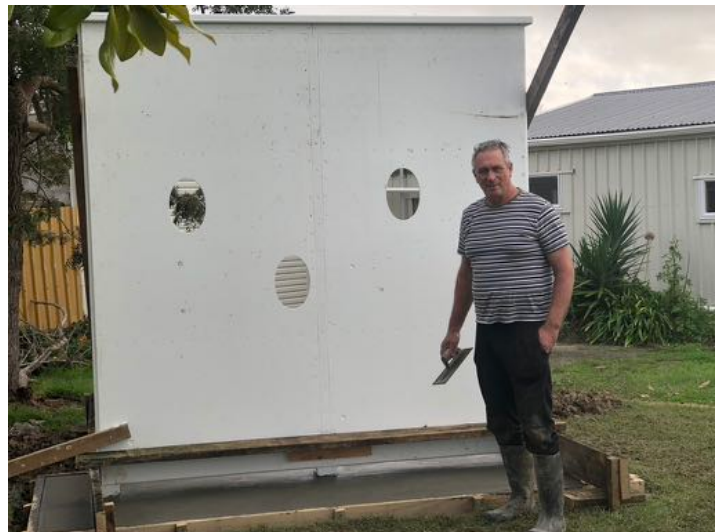
Tony King who did all the carpenter and concrete work
